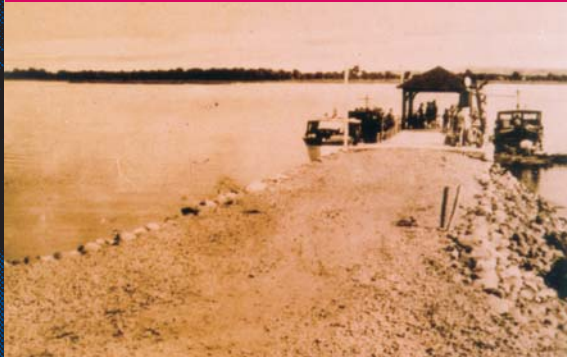
The original Government Dock was made of limestone and gravel.
